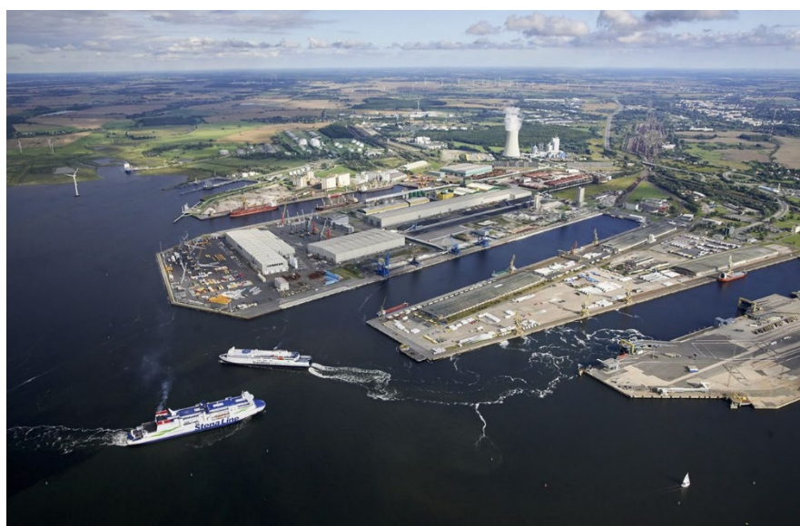
View of the port of Rostock where the green hydrogen plant is to be built Copyright: Rostock Port GmbH
